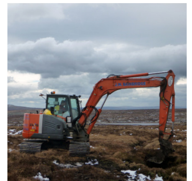
Reprofiling © North Pennines AONB Partnership
