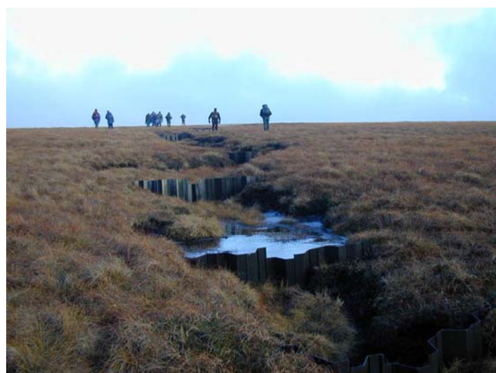
Figure 9. Gully blocking in narrow gullies using plastic piling
