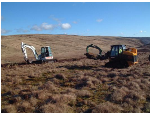
Drain blocking at Lake Vyrnwy using heather bale and peat dams
