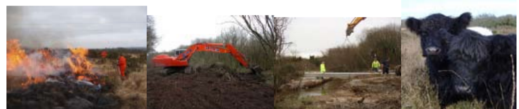
(1) Controlled burning (2) track clearance (3) vehicle bridge installation (4) project Belted Galloways
