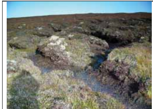
Figure 78. T4 erosion hagg
