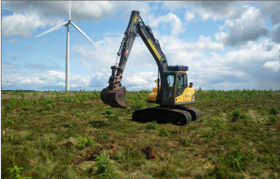
Photo F3: Excavator in the process of cross-tracking
