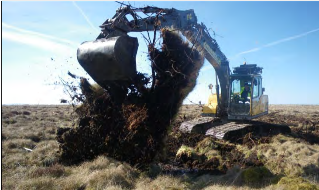
Photo F1: Stump being flipped over during the ground-smoothing process
