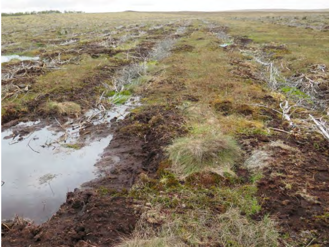
Photo G3: Brash crushing and furrow blocking within old felled to waste plantation at Dyke, Forsinard using extra-wide tracked excavator.
