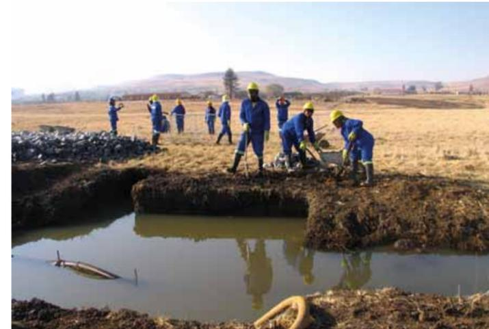
A Working for Wetlands team busy constructing a gabion weir (purpose to arrest erosion and lift up the watertable) in the Wakkerstroom mire, South Africa.
