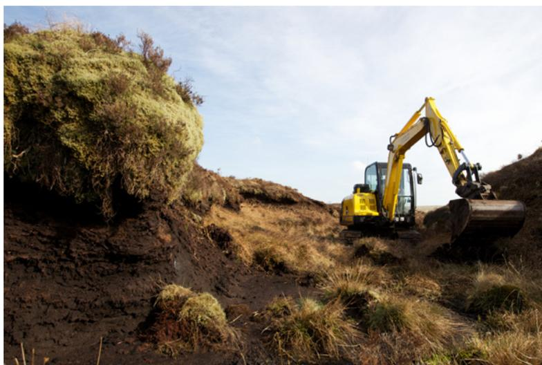
*An excavator carrying out reprofiling work as part of restoration. Restoring our peatlands is vital for achieving net zero in the UK, but if it is done to mitigate for the carbon emissions associated with the development these savings cannot be included as a net gain in the national accounting. © Montgomeryshire Wildlife Trust*
