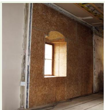
Figure 10: Insulating board 'Typha board' made from reedmace ©Typha Technik
