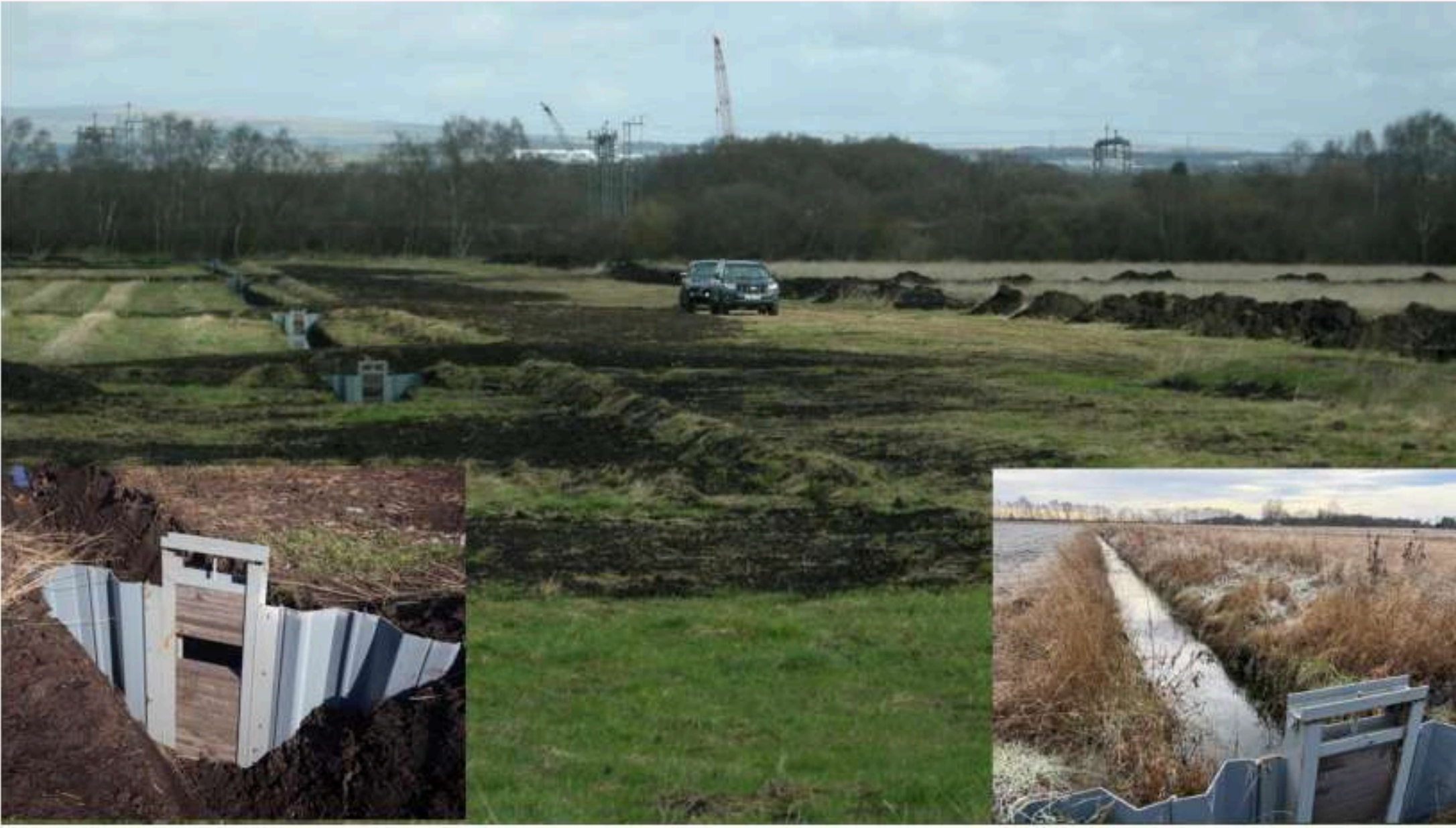
Capital works including deep trench bunding, cut-off ditches, water retention ponds and sluice gates to control in-field water levels
