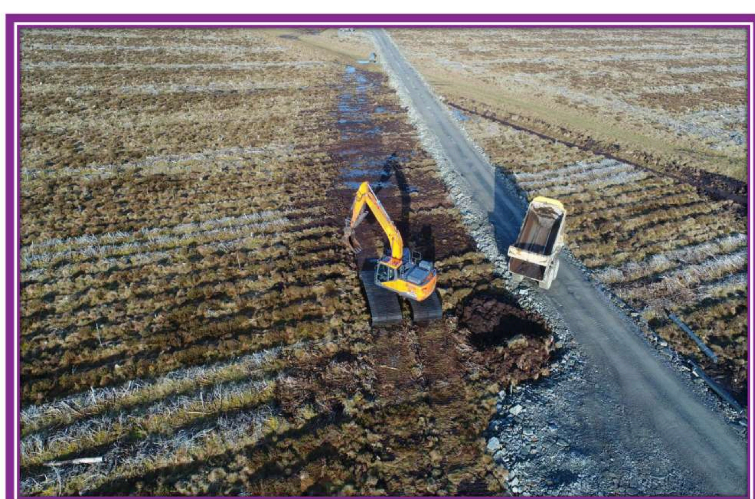
Picture 1: April 2024 – during reinstatement operation
