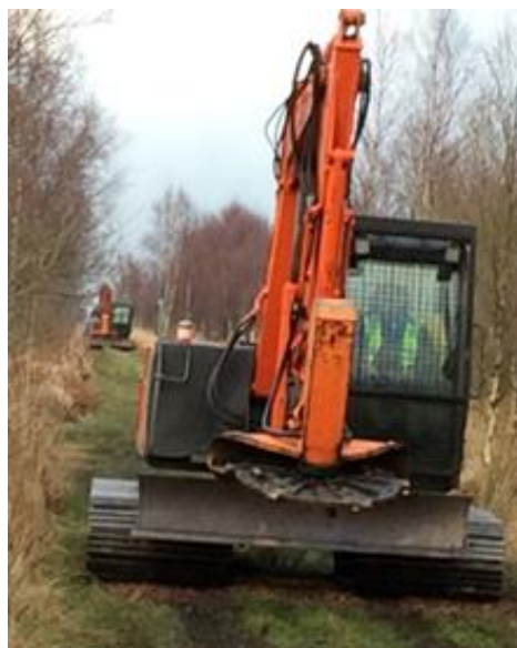
Excavator flail, Thorne. ©Ed Brightman
