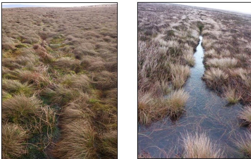
Figure 4: A reprofiled grip on Kelber moor (left) and a non-reprofiled grip on Hardcastle moor (right), both completed in March 2014.
