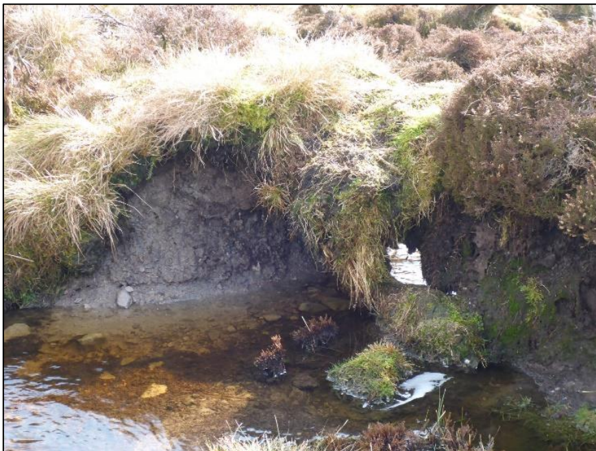
Figure 6: Eroded peat dam on The Preserves, 2017
