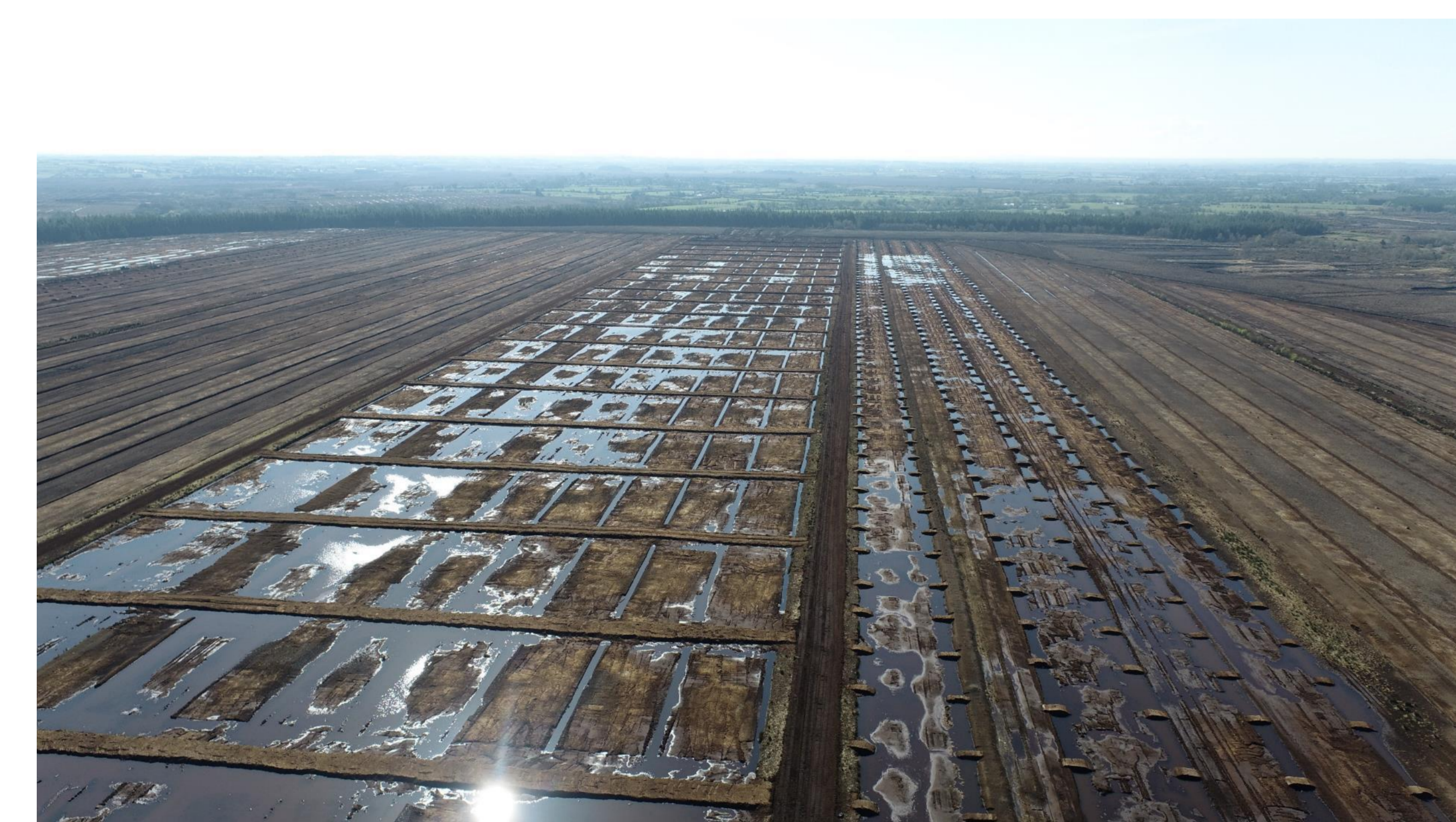
Castlegar Bog – cell bunding to re-wet peat across a slope. Some trial drain blocking on the right side.
