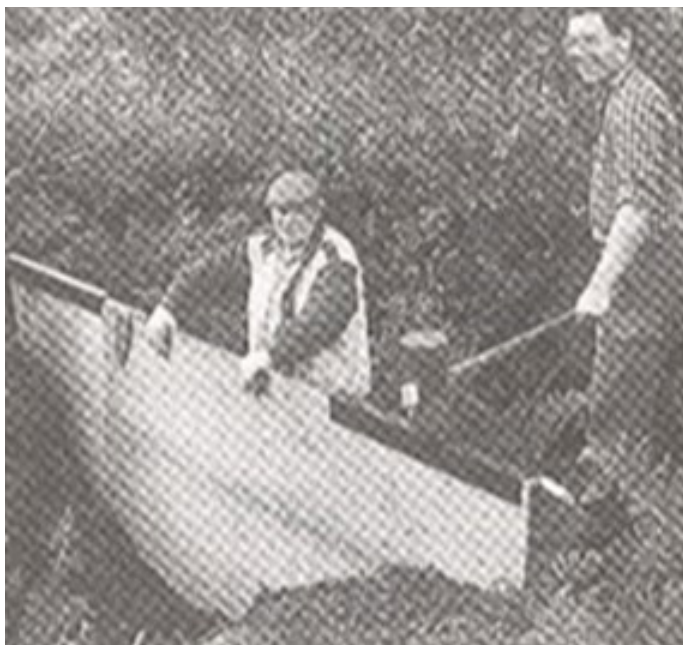
Figure 82 Hammering in a ply sheet dam. Note, the C-bar and use of rubber maul. © Stuart Brooks
