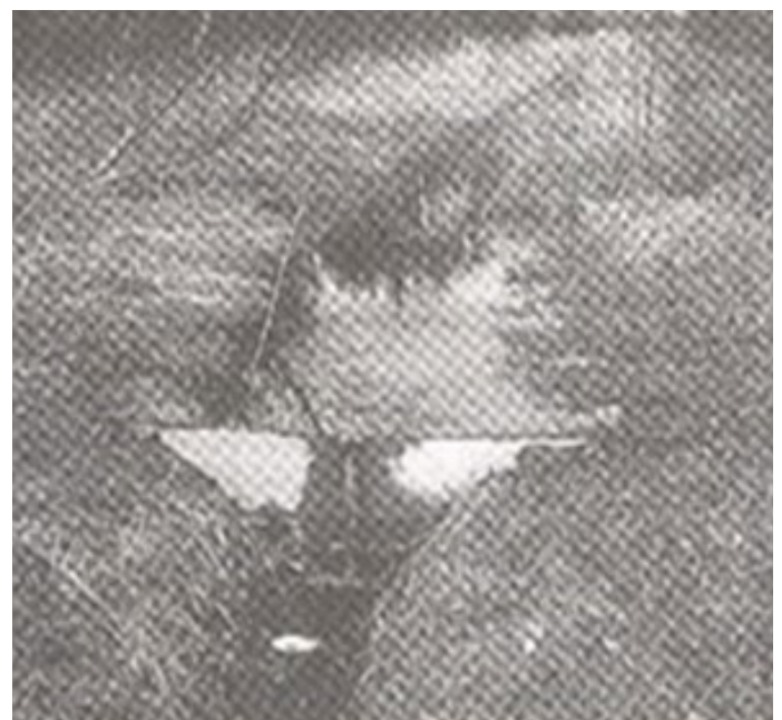
Figure 81 A plywood dam is prone to rotting at the air/water/peat interface. If the water level can be maintained at the bog surface and Sphagnum quickly recolonised, rotting is reduced © Stuart Brooks
