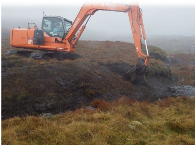
Figure 131 Reprofiling and turving eroding gullies, showing the steep-sided eroded edge to the right of the excavator bucket and the gently sloping and turved edge to left of the bucket © Yorkshire Peat Partnership
