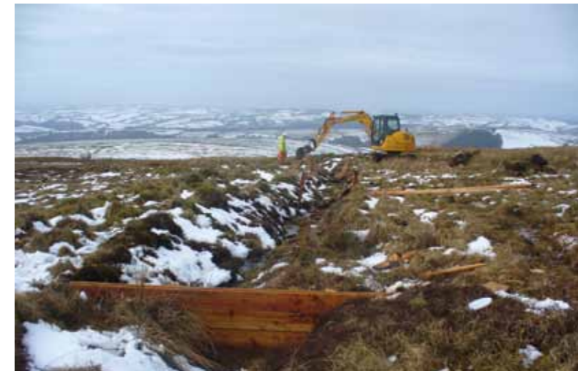
Blocking with wood, North Twitchen, Devon 2009 © Exmoor Mires
