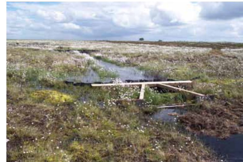
Effective plastic piling dam at Blawhorn © A McBride, McBride Habitats
