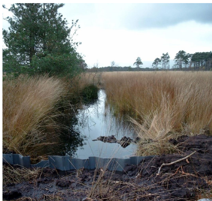
Figure 94 Large composite dam with plastic piling and peat on Foulshaw Moss SAC © Simon Thomas, Cumbria Wildlife Trust
