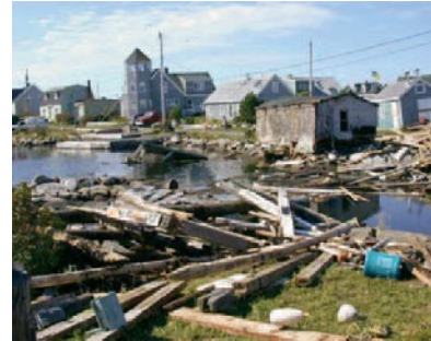
Hurricane Juan damage in Prospect, NS
