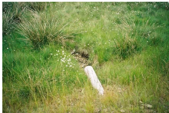
Figure 16 a and b Track across peat (cotton grass flush) to wind turbines at Ovenden Moor, West Yorkshire, showing use of sub-track drains and gravel to prevent erosion
