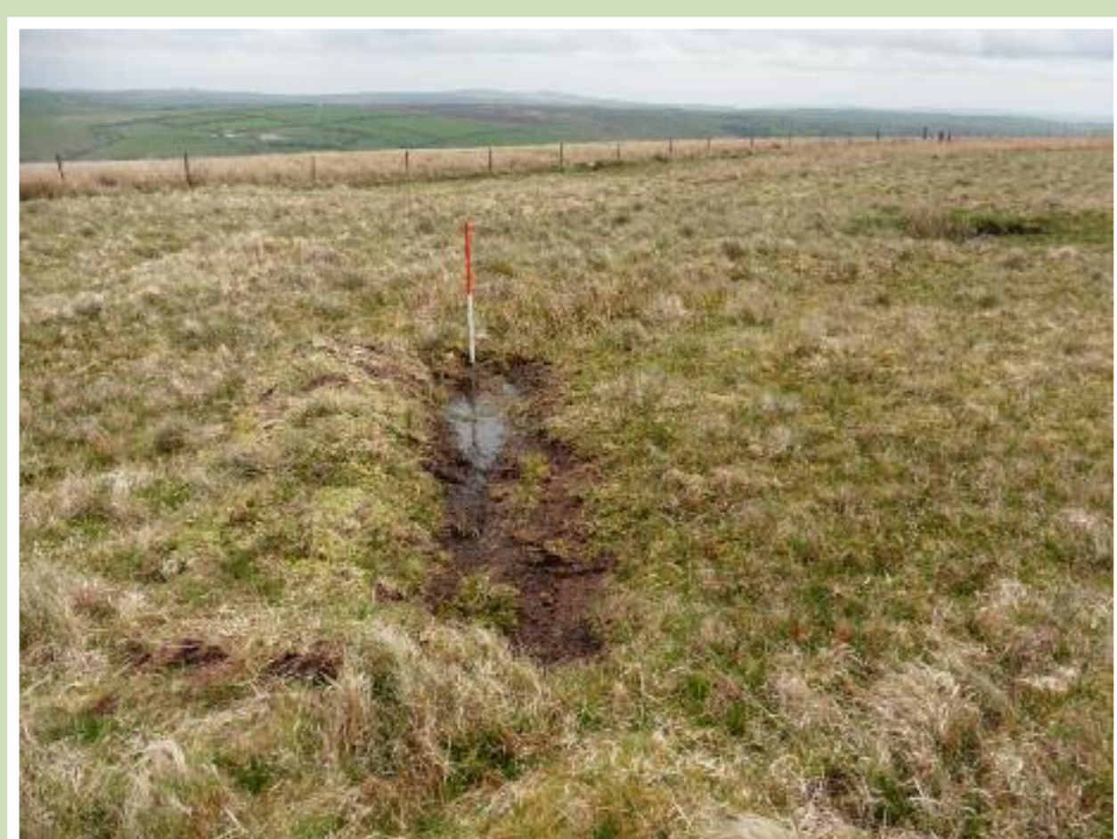
Left: Block made of peat to block exit point of a peat cutting.
