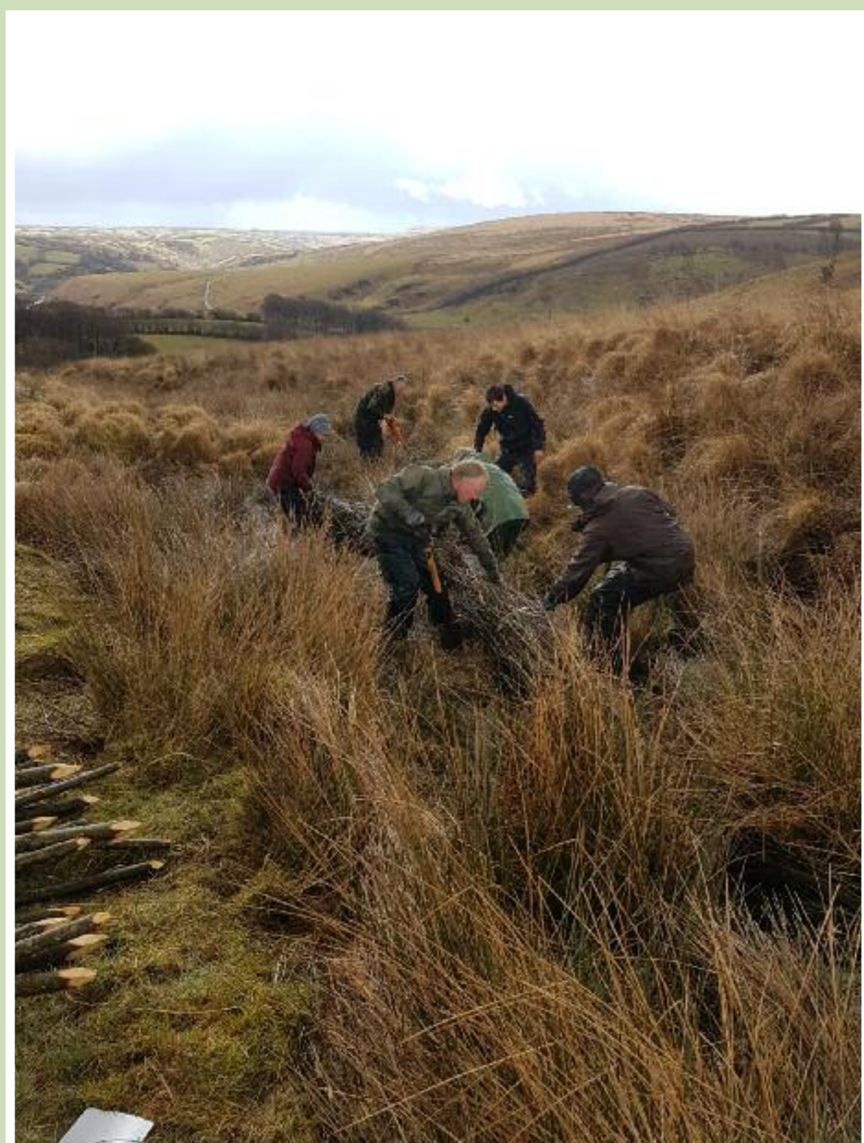
Below: Willow fascines installed in the gully.
