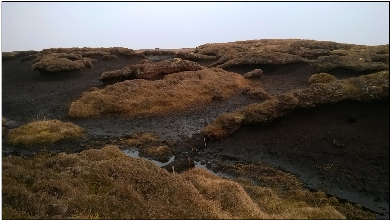
Gully bund on Shetland comprising salmon smolt net rolled-up, keyed into peat and pegged-in
