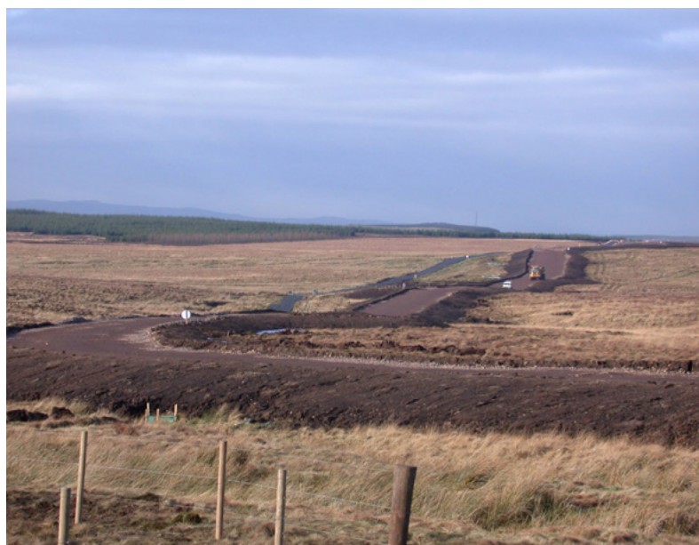
Roads and tracks constructed across peatlands can result in the excavation of peat but also lead to a severe impairment of the hydrological functioning of the landscape. © Ian Thomas SEPA
